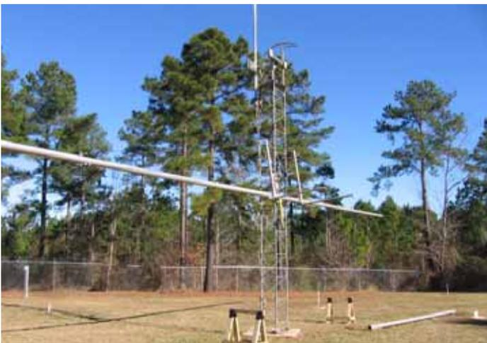
Each riser was 15ft of 2" x 1/8" wall tubing. We put an antenna at the top and bottom of each riser. Each riser has a stiff arm to support trusses. The individual trusses were spaced 17ft apart for a total length of 51ft on the boom. That left us 4.5ft on each end to attach the various trusses and for tie down ropes.
